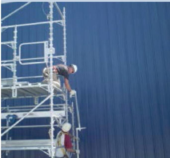
**2** Person below then raises lower end connector attaching it to appropriate height where top bar becomes level.
