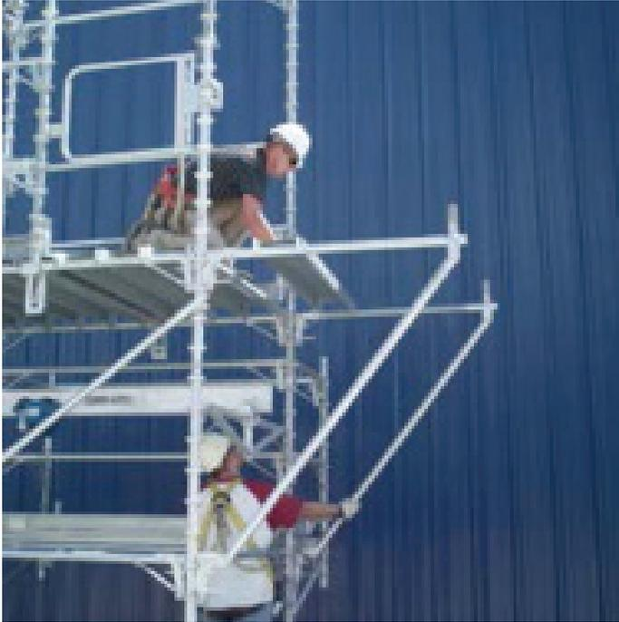
**5** Once decking is completed, install two (2) eight-cup verticals for handrail posts.
