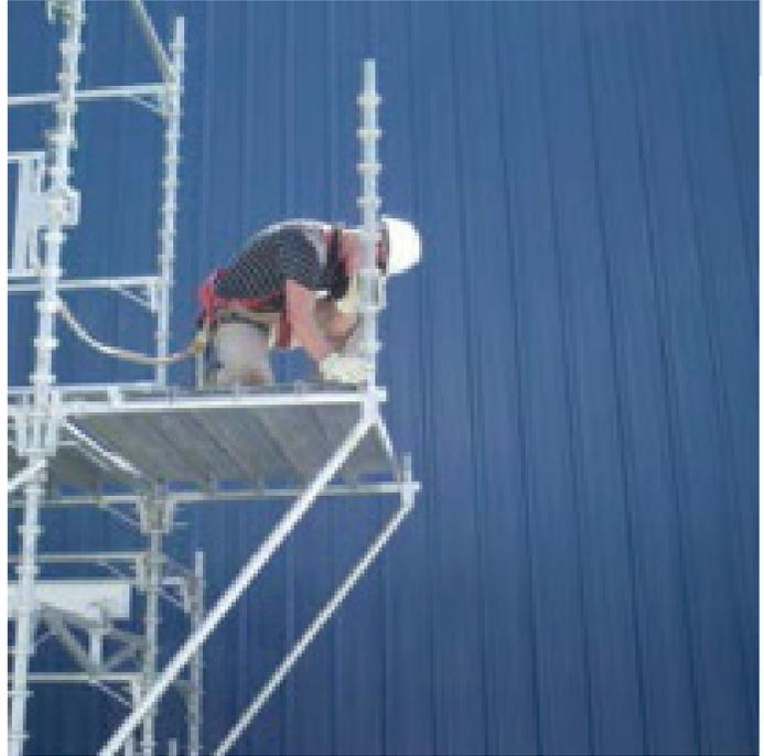
**6** Complete by enclosing side rails (same length as bracket), then end rails (same as deck length) and finally adding the toe boards.
